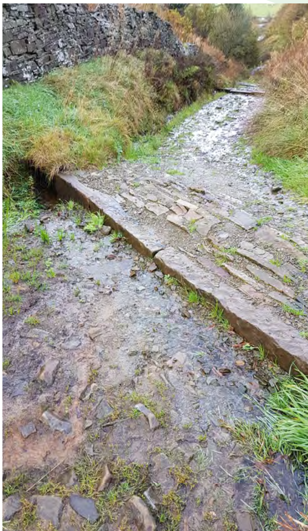
Cross drain ©Terra Firma Ltd
