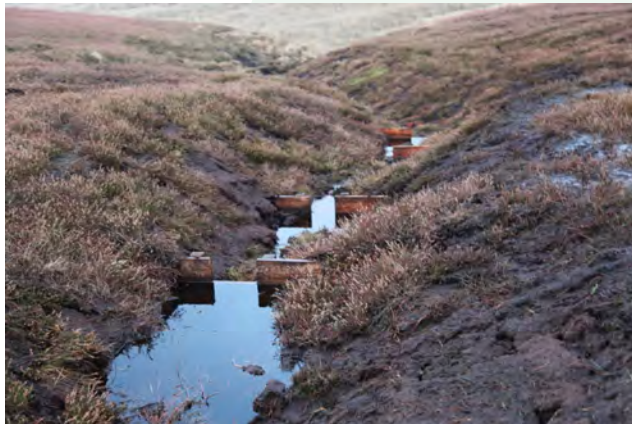
Anglezarke wooden dams and reprofiling ©Forest of Bowland AONB
