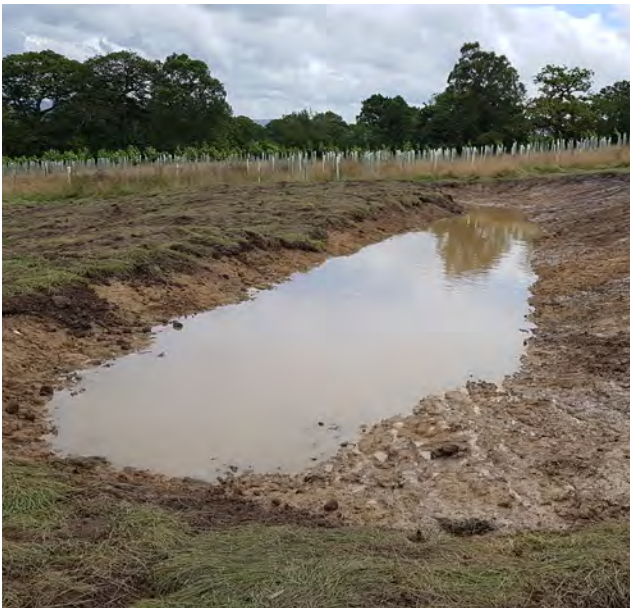
Detention Basin (Lower Knotts) © Ribble Rivers Trust
