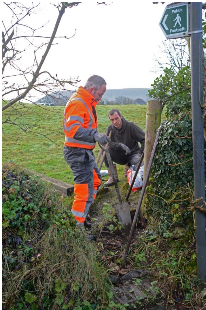
Pendle Lengthsman repairs
