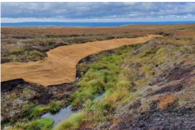
Geo-textile laid to protect the gully side, ready for seeding & brash; revegetation on site 2 years after the original work
