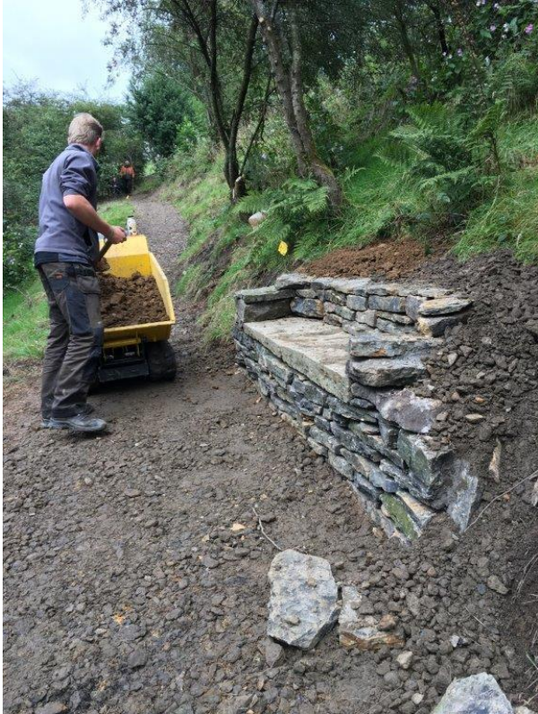
The new stone benches installed....
