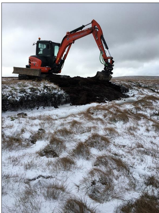
Re-profiling of peat hags and installation of timber dams to reduce run off, loss of peat soil and gullying
