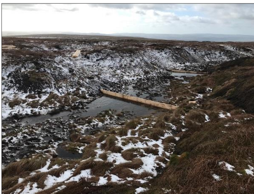
Re-profiling of peat hags and installation of timber dams to reduce run off, loss of peat soil and gullying
