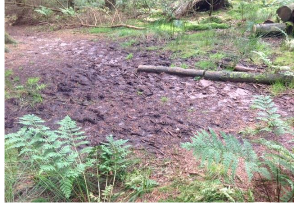
Route 6: potential permissive route link, drainage channel needed
