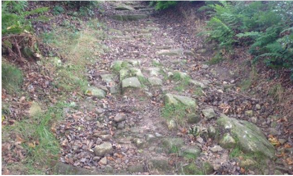
Route 2: Poor surface in places
