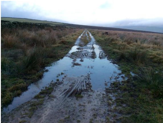
Coal Pit Lane, wet sections, looking East
