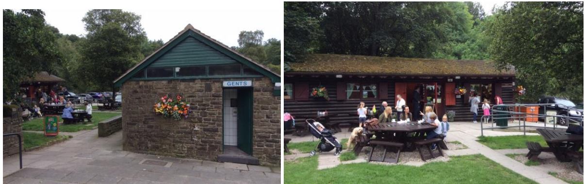
Figure 8: Toilet and cafe at Barley
