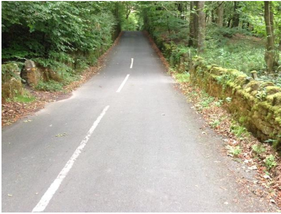
Route 5: Potential Crossing Point GR SD 772 364, Looking SW
