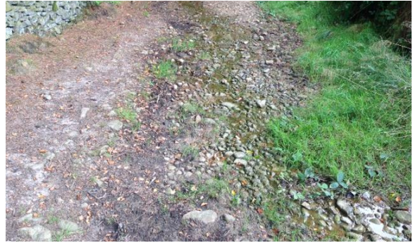
Route 2: Surface water due to insufficient/blocked drainage
