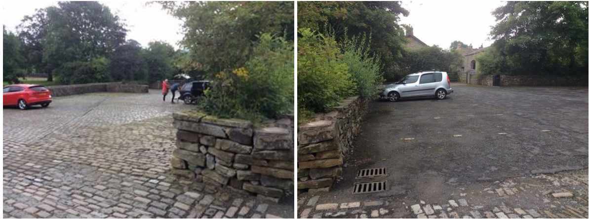
Figure 14: Downham Car Park
