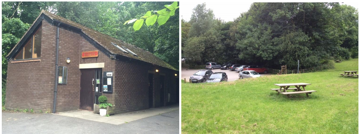
Figure 19: Spring Wood toilets and carpark
